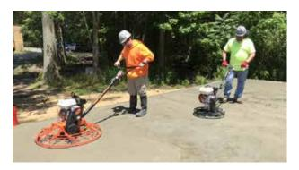
The F24 EDGER TROWEL is ideal for jobs that require a lightweight, highly maneuverable, professional finishing tool. This specialty finishing power trowel allows professional results even when confined areas or weight restrictions leave other machines standing idle. Perfect for edging in the tightest spaces, the F24 Walk Behind Power Trowel is always ready when needed.
